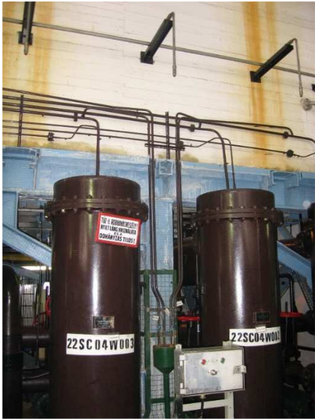
Figure 2.1.4-2: Water mist extinguishing equipment
