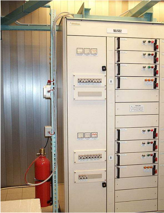
Figure 2.1.4-3: Local gas extinguishing system in Electrical Building
