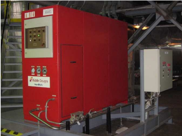
Figure 2.1.4-2: Water mist extinguishing equipment
